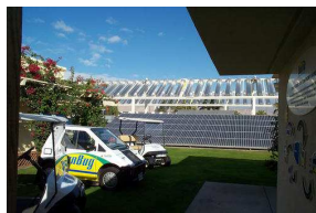
Solar-powered electrolysis system at SunLine Transit Agency
